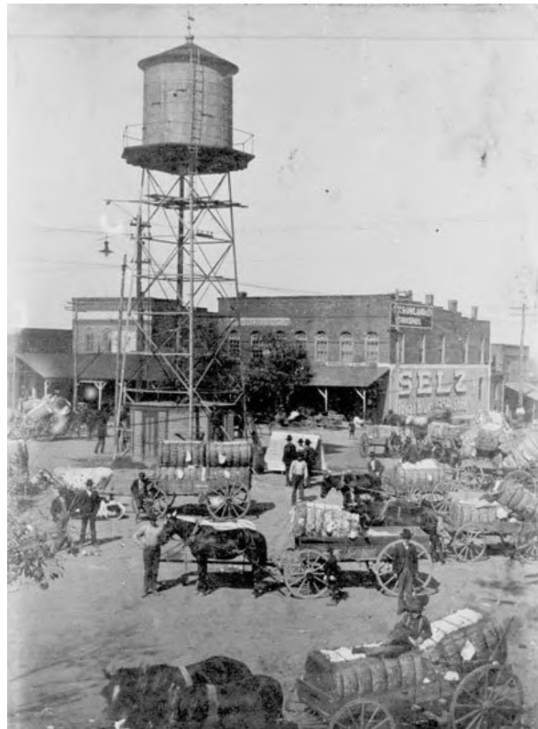
Square with water tower - B. M. Long Photograph Album: donated by Aubrey Jones: Special Collections: SUWG
